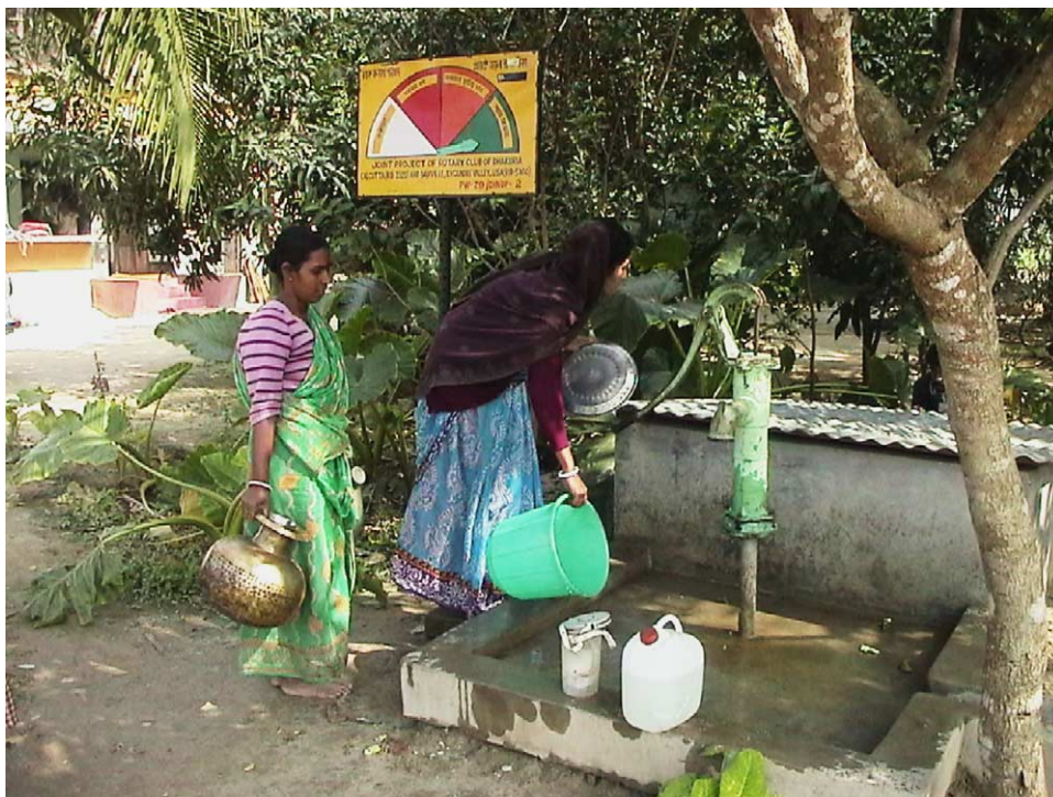
Fig. 1. Newly installed shallow dugwell with hand pump extraction of water to replace tubewell with water arsenic concentration of 220 \mu\text{g}/\text{l} . Arsenic concentration in this dugwell was 6 \mu\text{g}/\text{l} , but concentrations in such dugwells may be in range from 2 to 50 \mu\text{g}/\text{l} .
